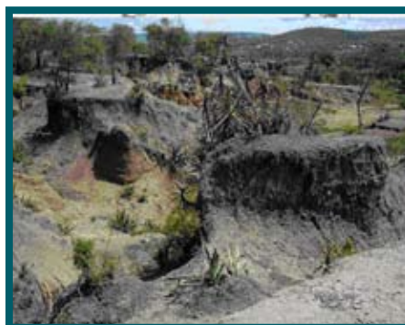
Land degradation due to surface runoff
