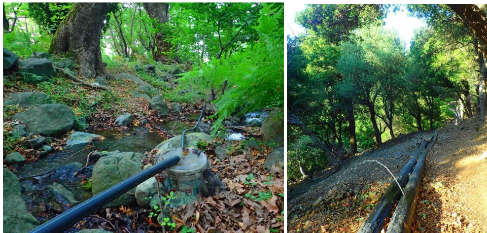
Figure 4: Bucket filter; Figure 5: Overpressure hole in PVC pipe.
