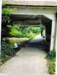
Missing railing under the bridge
