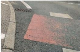
Curb stone is not comfortable, bad conditions of painting mark (worn out) / accident hotspot
