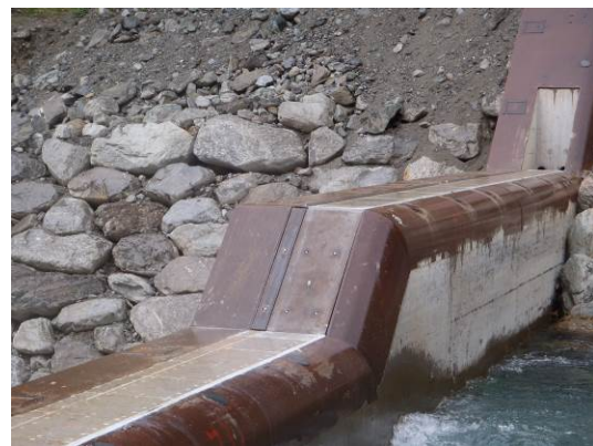
Figure 7: Detail of the equipped check dam (during installation in June 2013).
