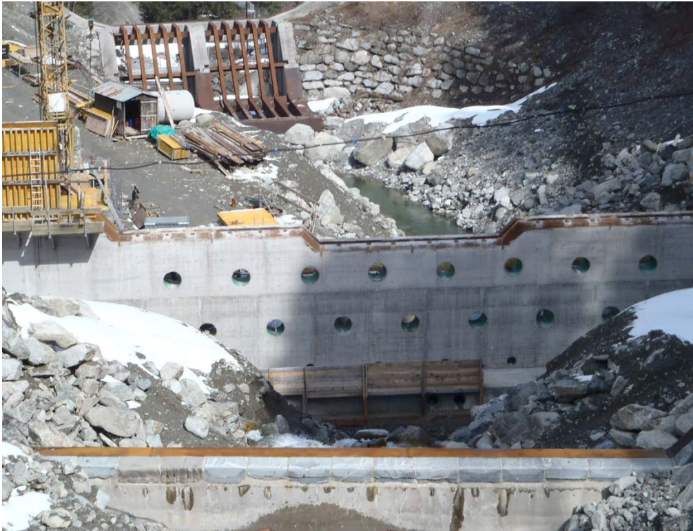
Figure 1: Structured check dam prepared for installation of the measuring system.
