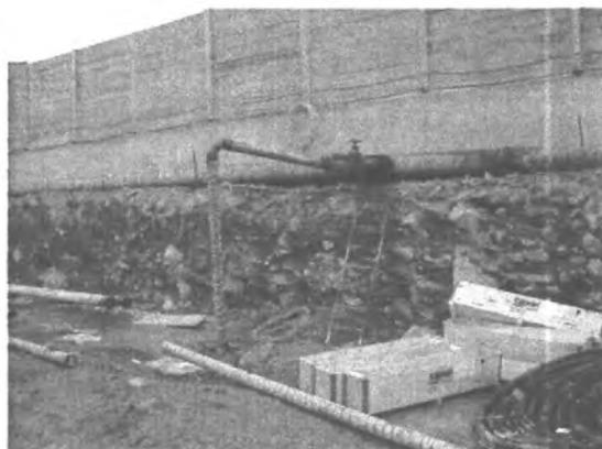
Abb. 10: Jet-grouting Wand, Anker, Brunnen
