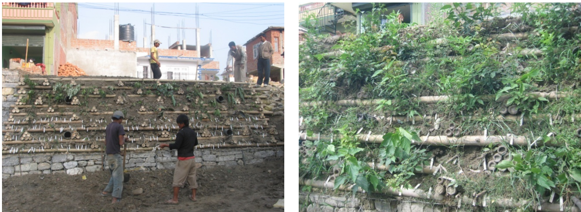
Figure 4: The vegetated bamboo crib wall just after construction (November 2006) and after one year of construction (Kusunti, Lalitpur, November, 2007)
