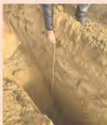
Fig. 2 Test pit no. T1 in Hollabrunn, Lower Austria, depth approx. 3m
