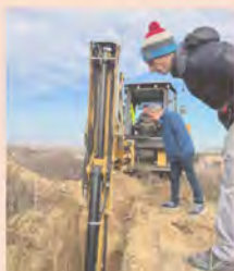
Fig. 1 Digging of test pit in Hollabrunn, Lower Austria
